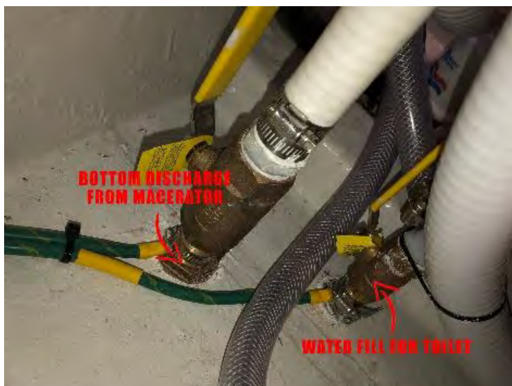
Intake/Fill Valve in the "OPEN" Position
