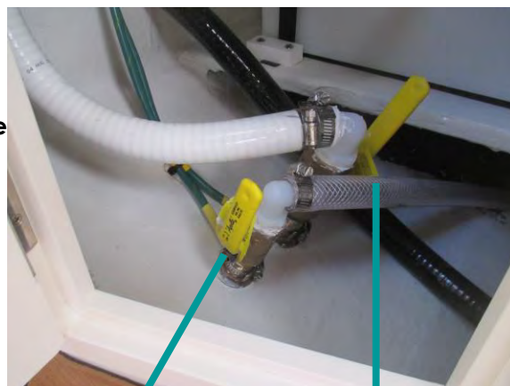
Intake Valve (open)
